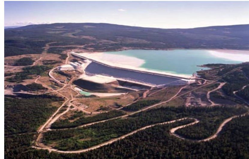
The L-L embankment of the Valley impoundment The Highland Valley Copper Mine is located just outside the town of Kamloops in British Columbia, Canada. The mine produces copper (435,000 tons in 2003) and molybdenum (6405 tons in 2003) concentrates. The tailings pumped to the Valley Impoundment in 2003 were 48.5 million tons.
